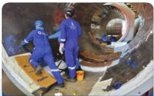
WHRU Exhaust Insulation
