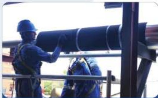
Cellular Glass Insulation
