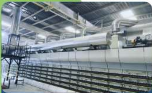
High Temperature Insulation & Jacketing for Process Plants
