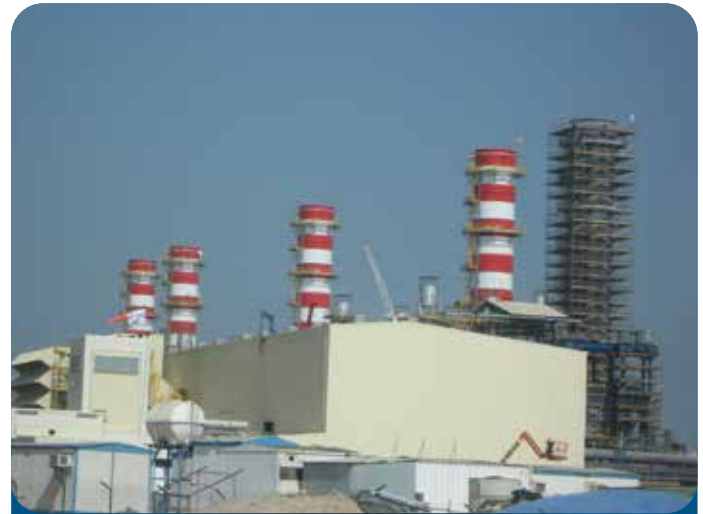
Gas Turbine Exhaust Stacks
