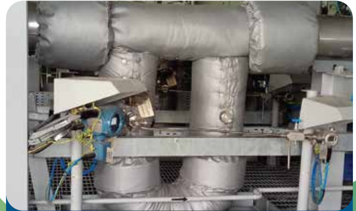
High Temperature Removable Thermal Jackets for Petrochemical Plants
