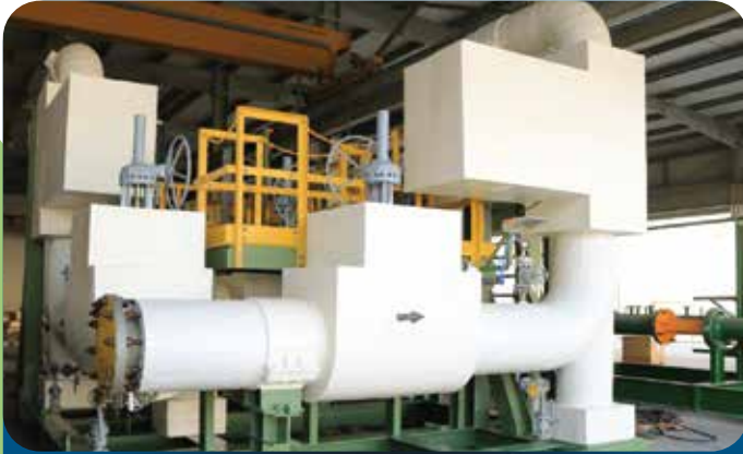
Cryogenic Insulation & GRP Lamination for Ammonia Metering Skids
